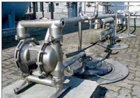
1 1/2" diaphragm pump installed in a chemical process to transfer chloride methylene
